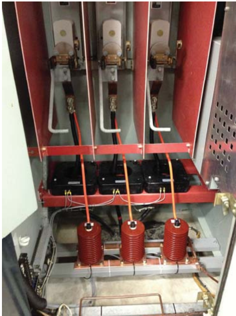
Fig. 14 An example of a 3 pole HSGS retrofit
